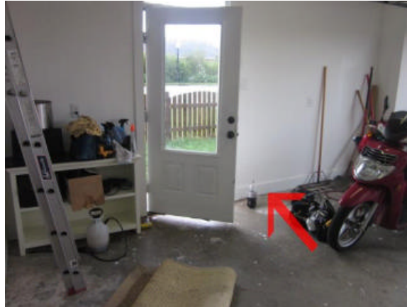
Water entering into the side garage door and vicinity.
